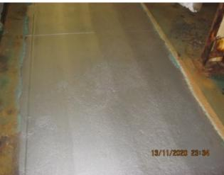
Cleaning and preparation resulting in a clean blasted deck with no dust or debris to clean up
